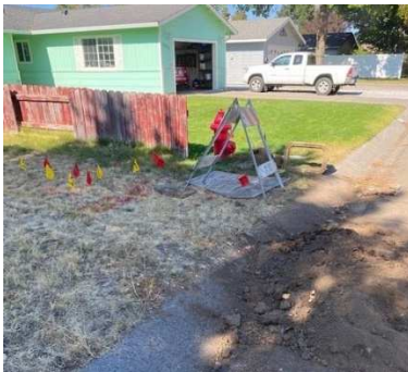
WhiteHawk Construction installing new radio read meters
