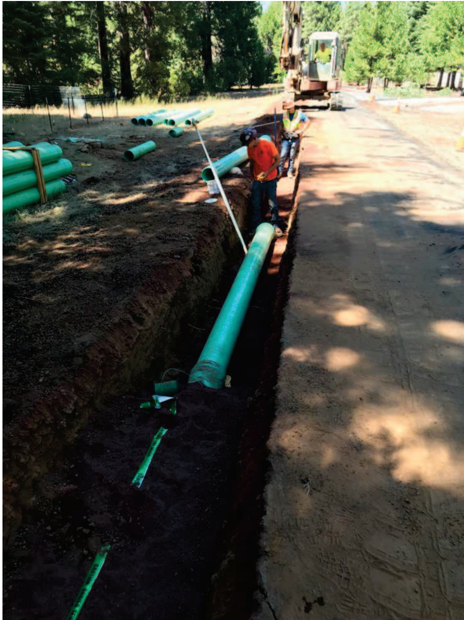
Photo 3 – Sapphire Way Sewer Main Replacement
